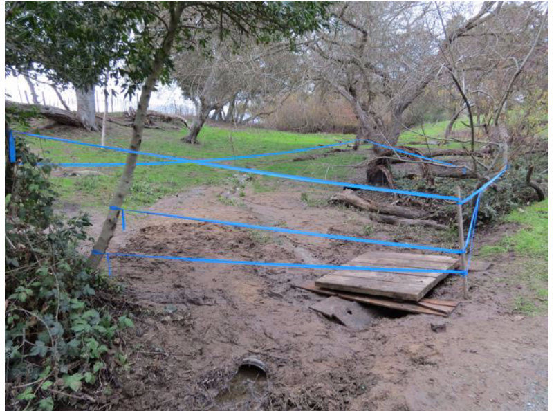
Damaged understory and drainage at Pinto Lake County Park. Photo: Bernadette Ramer
